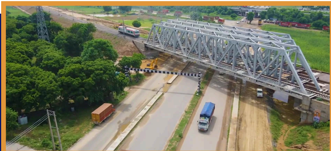
Major Bridge Over Pataudi Road on Patli-Manesar-MSIL Rail Link
