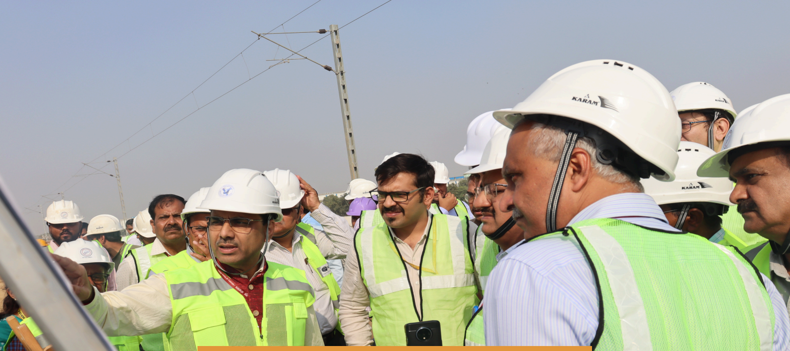
NR Safety Team inspection of Patli-Manesar-MSIL Rail Link
